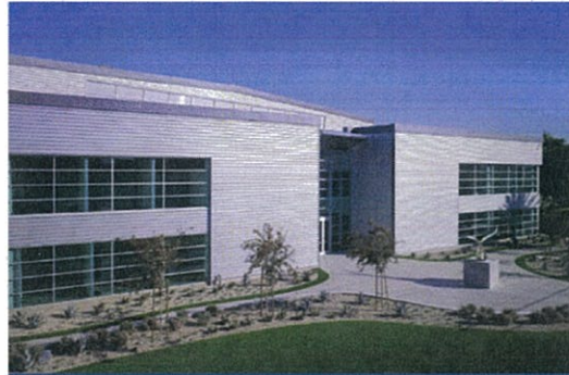
SUN SPOT: Hangar 25 at Bob Hope Airport in Burbank, Calif., uses solar energy to power aircraft undergoing maintenance.
